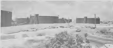
At left is the new refinery wall west of Lago Heights Gate (No. 8). View is from Lago Heights hill looking southwest. Picture below (r to l) shows part of well from Gate No. 1 in northern direction.
